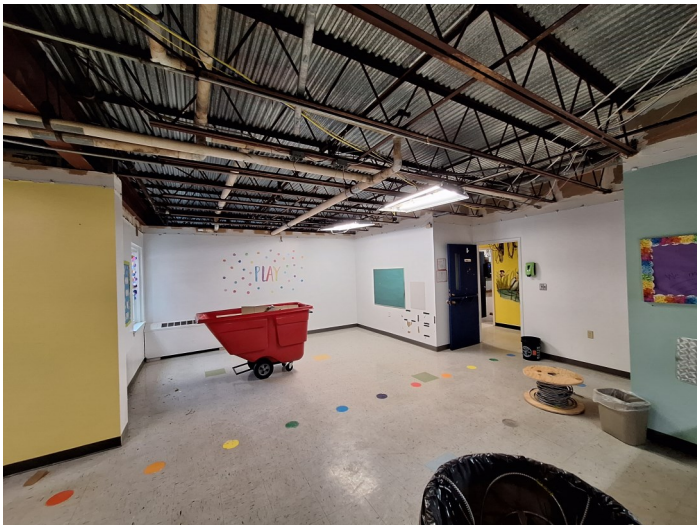
Classroom grid and tile removed
