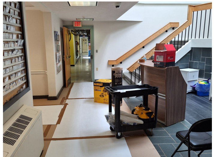
Main entrance flooring protected.
